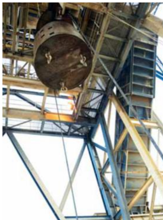
With the 'owner's team' in charge, Kibali achieved a sinking rate for the vertical shaft 50% higher than the industry norm, reaching the bottom at 751 metres three months ahead of schedule.
